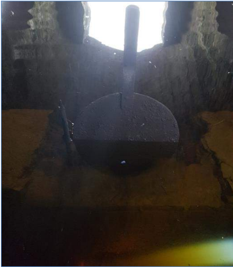
Photo 5 – Gate valve in Bay 6, rectangular ope below
