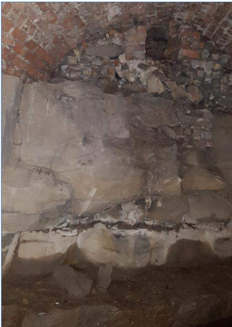
Photo 2 – End wall of Bay 1 constructed on limestone rock
