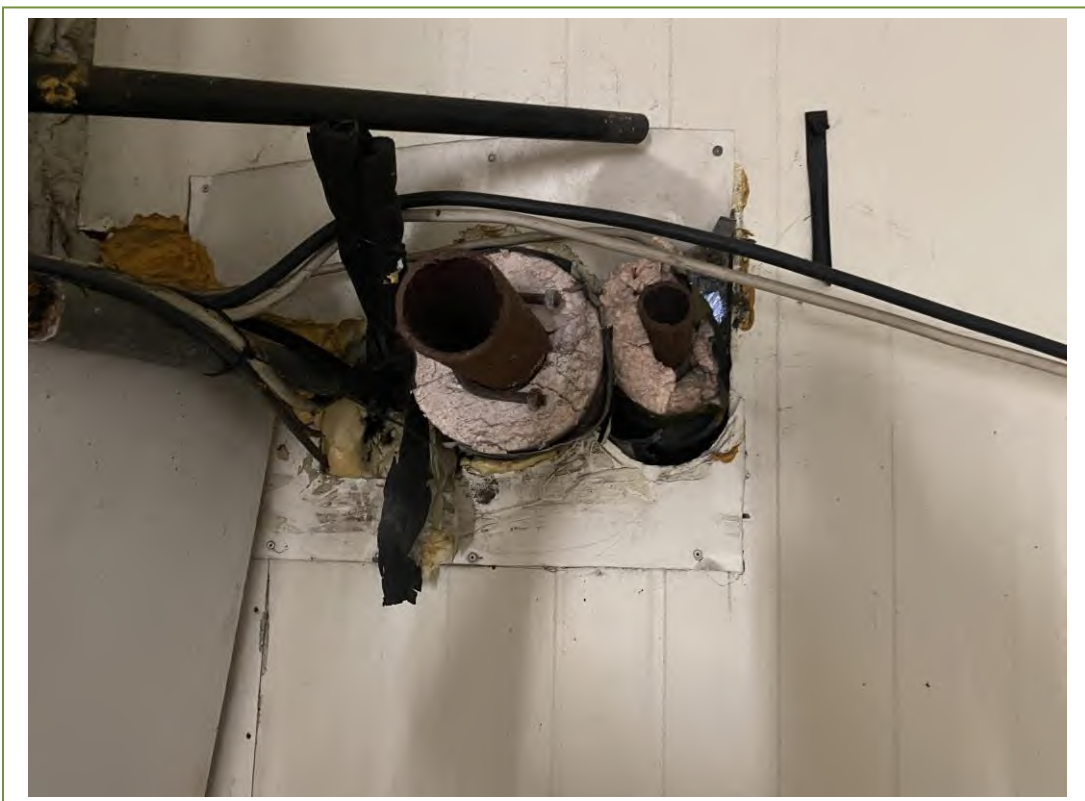
Pipework insulation sampled in building 5
