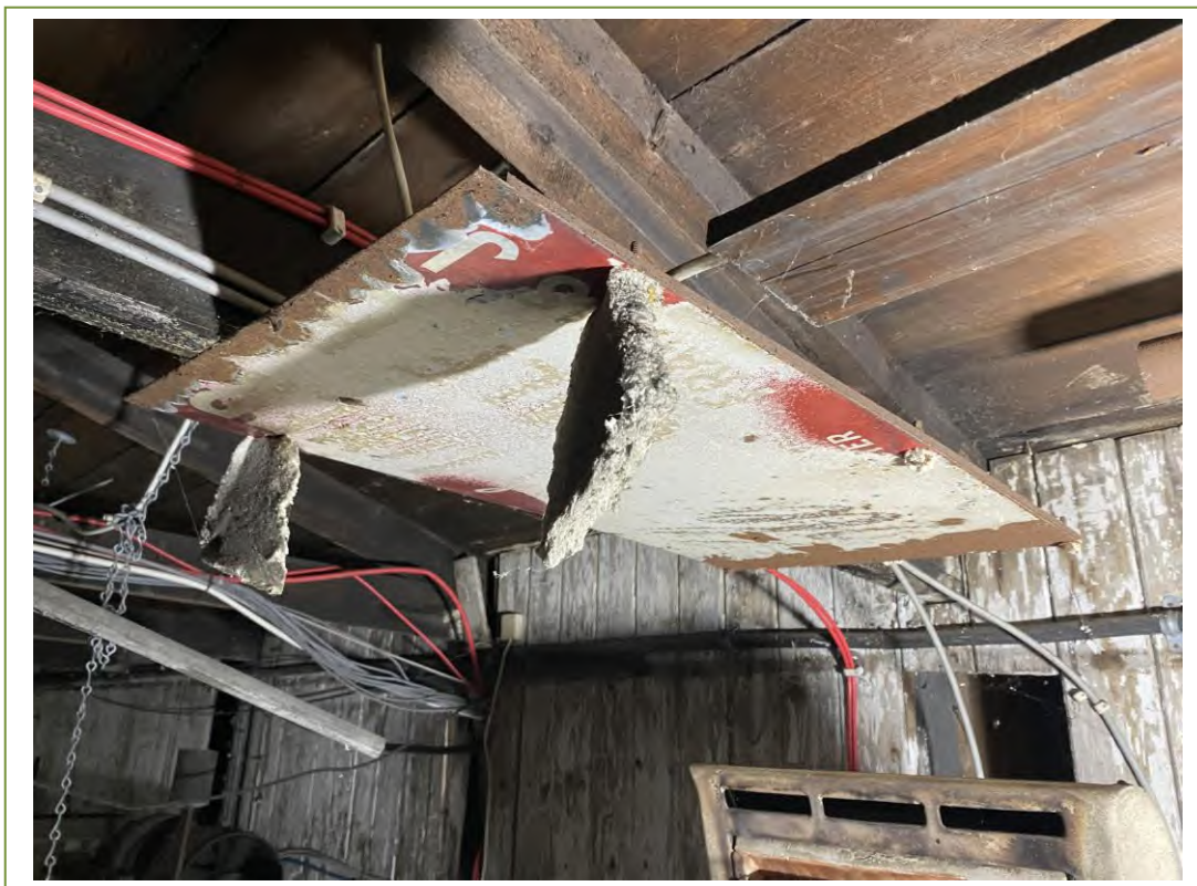
Closeup view of the remaining millboard on one of the panels over the heater
