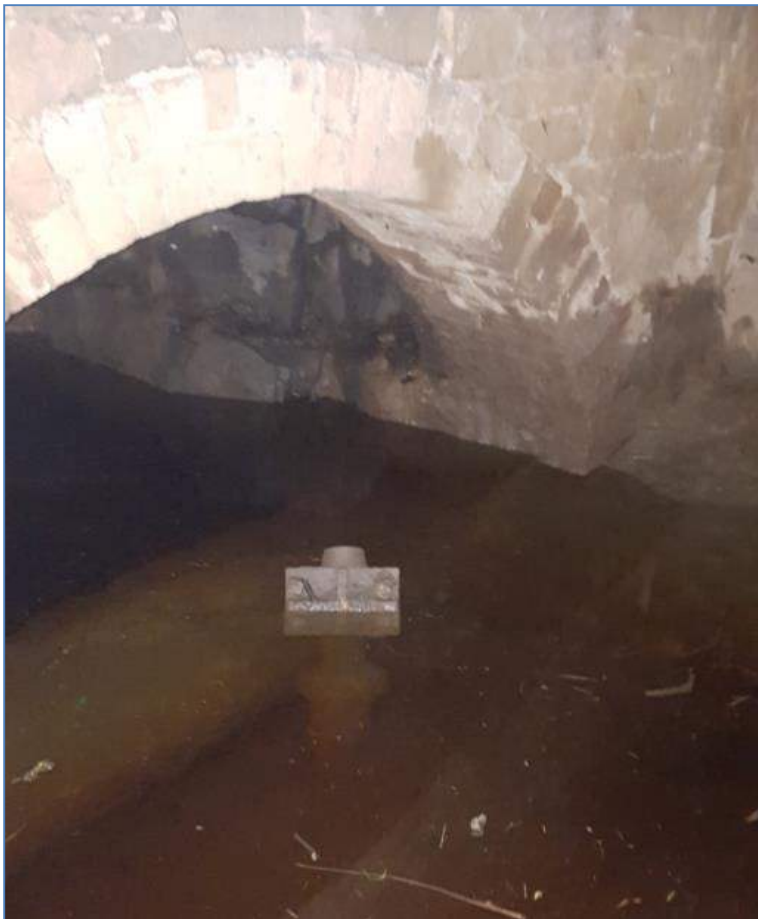
Photo 4 – Delivery pipe nozzle in Bay 4, pointed into Bay 3, submerged wall visible
